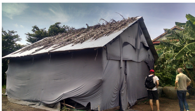
Figure 4. Mushroom house with a metal roof. The farmer has placed palm fronds on top in an attempt to regulate the temperature inside the house
