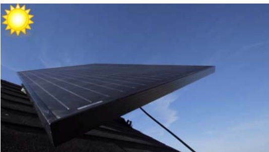
Fig. 2. Tracker in flat position (noon)
